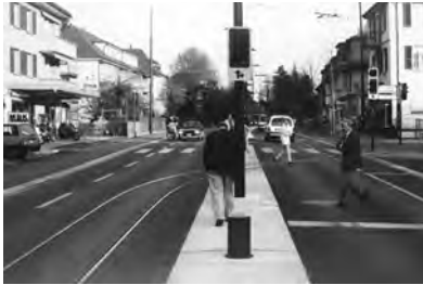
Two-stage crossings make it easier and safer for children to cross the road: they should be systematically provided at all the approaches to schools. Older people and those with reduced mobility would also benefit.
