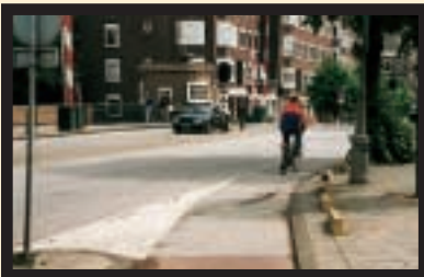
Cycle path ends smoothly where cyclists re-enter mixed traffic lanes.
